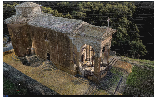
Fig. 2. View of the 3D reconstruction (photogrammetry and laser scanning) - SS. Crocifisso al Calvario Church
